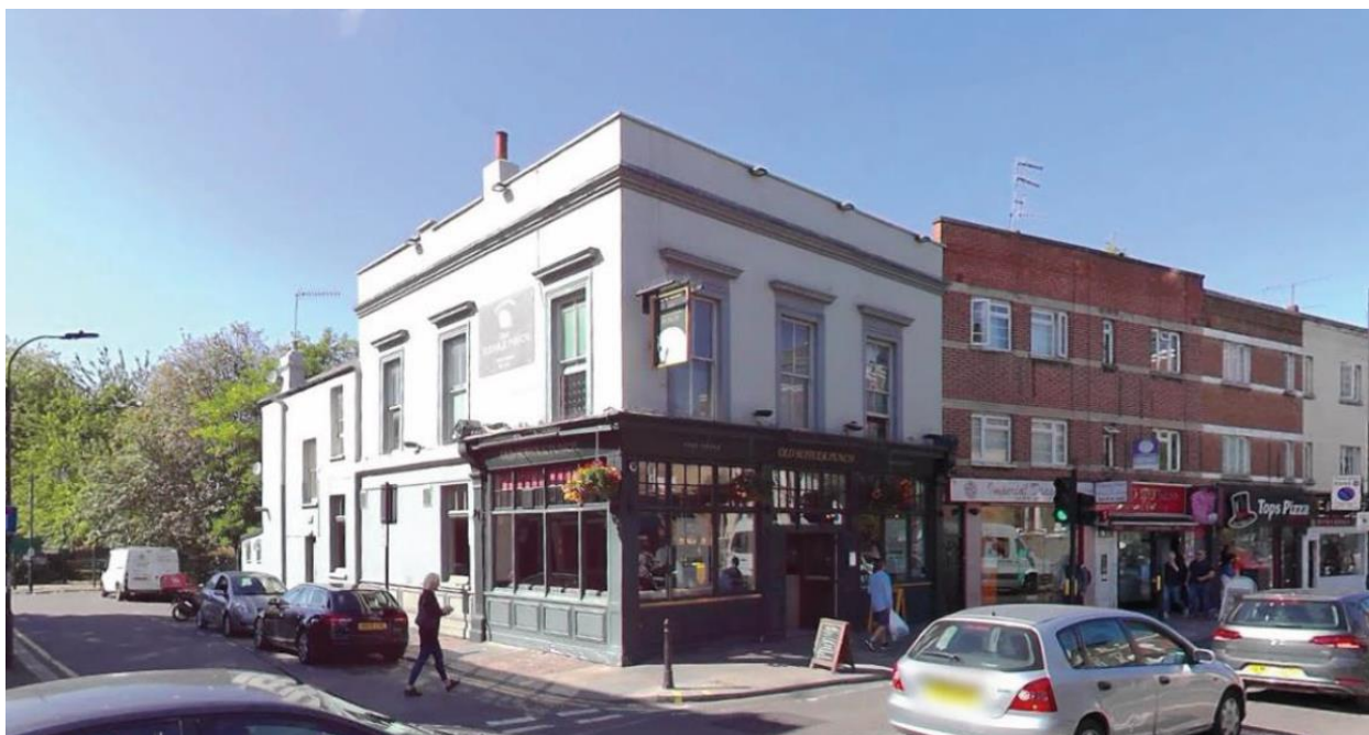
Figure 1 - site as existing, viewed from Fulham Palace Road
